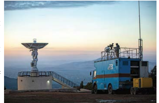
Ethiopian Multi-Satellite Ground Receiving Station
