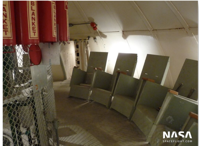
The Apollo "Rubber Room" at LC-39. A bunker is located 40 feet beneath the launch pad. Dome-shaped, built on springs and shock absorbers, to be used in the event of an imminent Saturn V explosion with workers at the pad.
