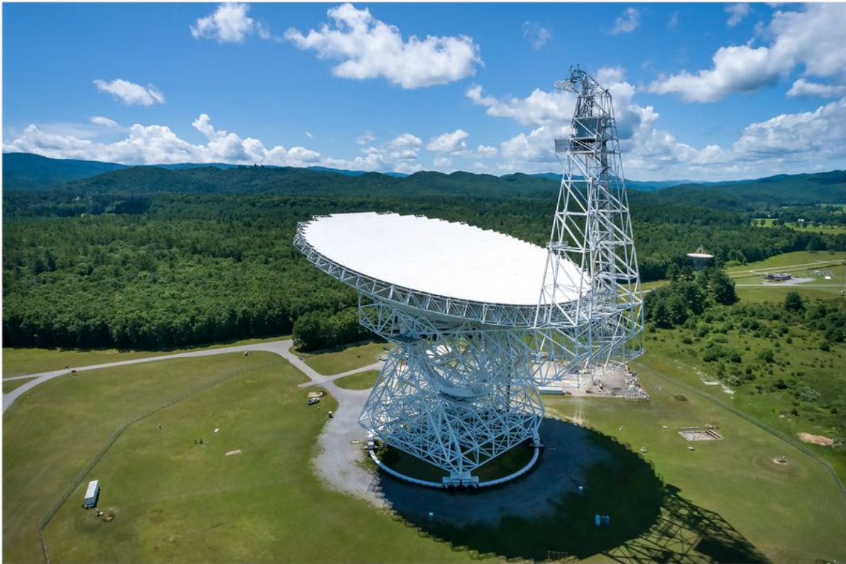
The Green Bank Observatory in West Virginia. Equipped with a motorized, football field-sized dish that seeks out celestial phenomena like pulsars, gas clouds, and distant galaxies. It is the world's largest steerable radio telescope!
